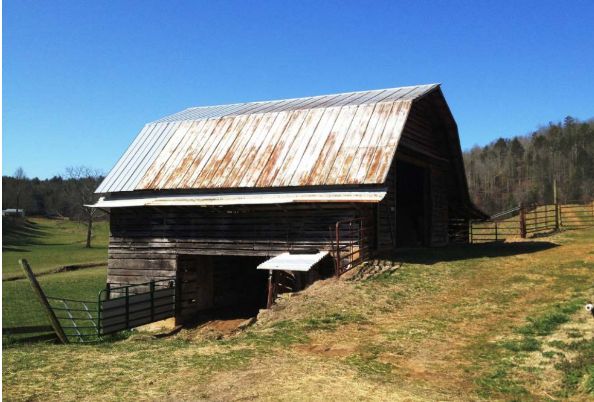
Barn, oblique front view to west
