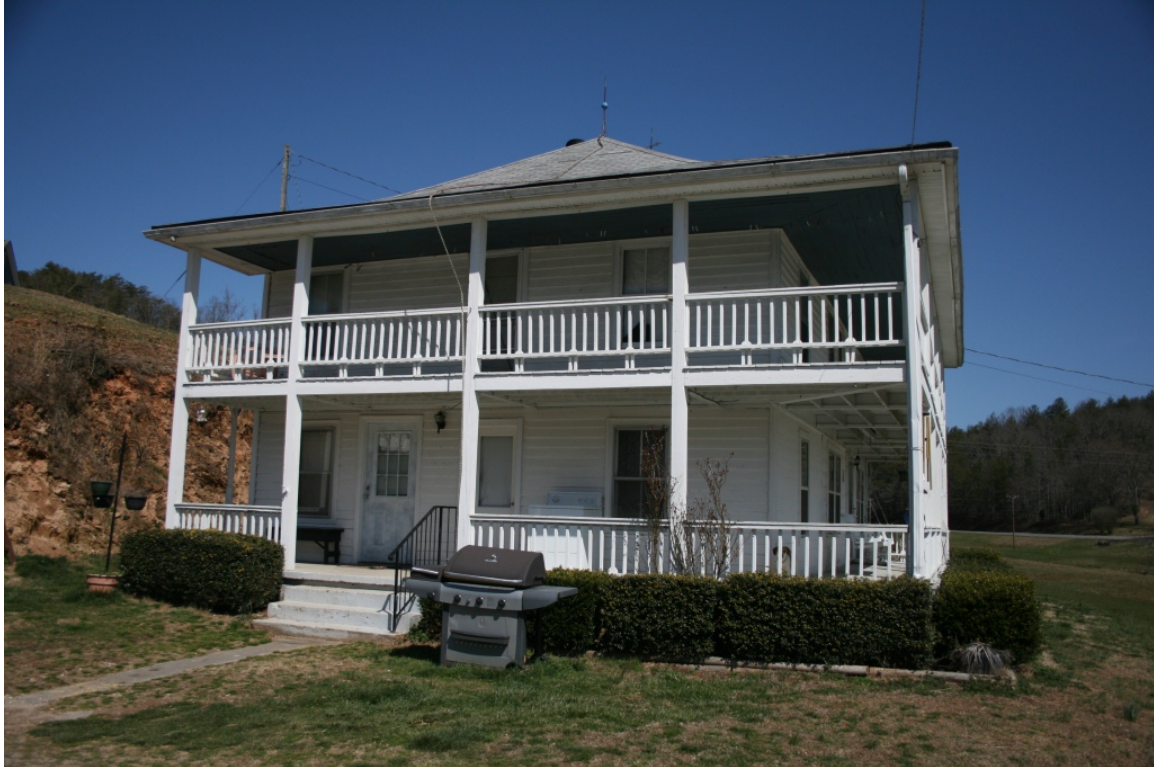
Hickey House, southwest elevation, view to north
