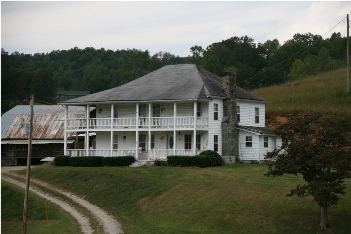
Hickey House (CE 117), 3845 NC Hwy 294, oblique front view to west
