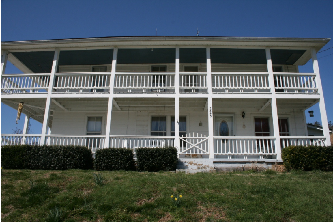
Hickey House, façade, view to northwest
