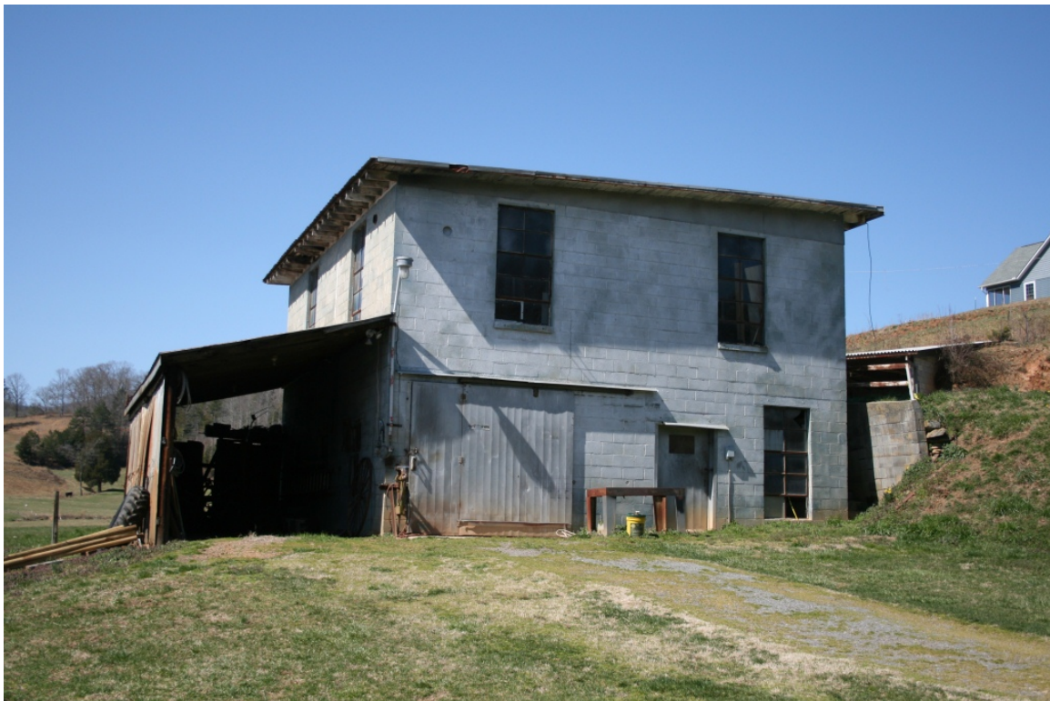
Sheet metal shop, east elevation, view to west
