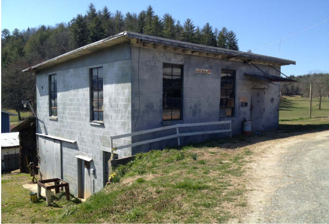
Sheet metal shop, oblique front view to southwest
