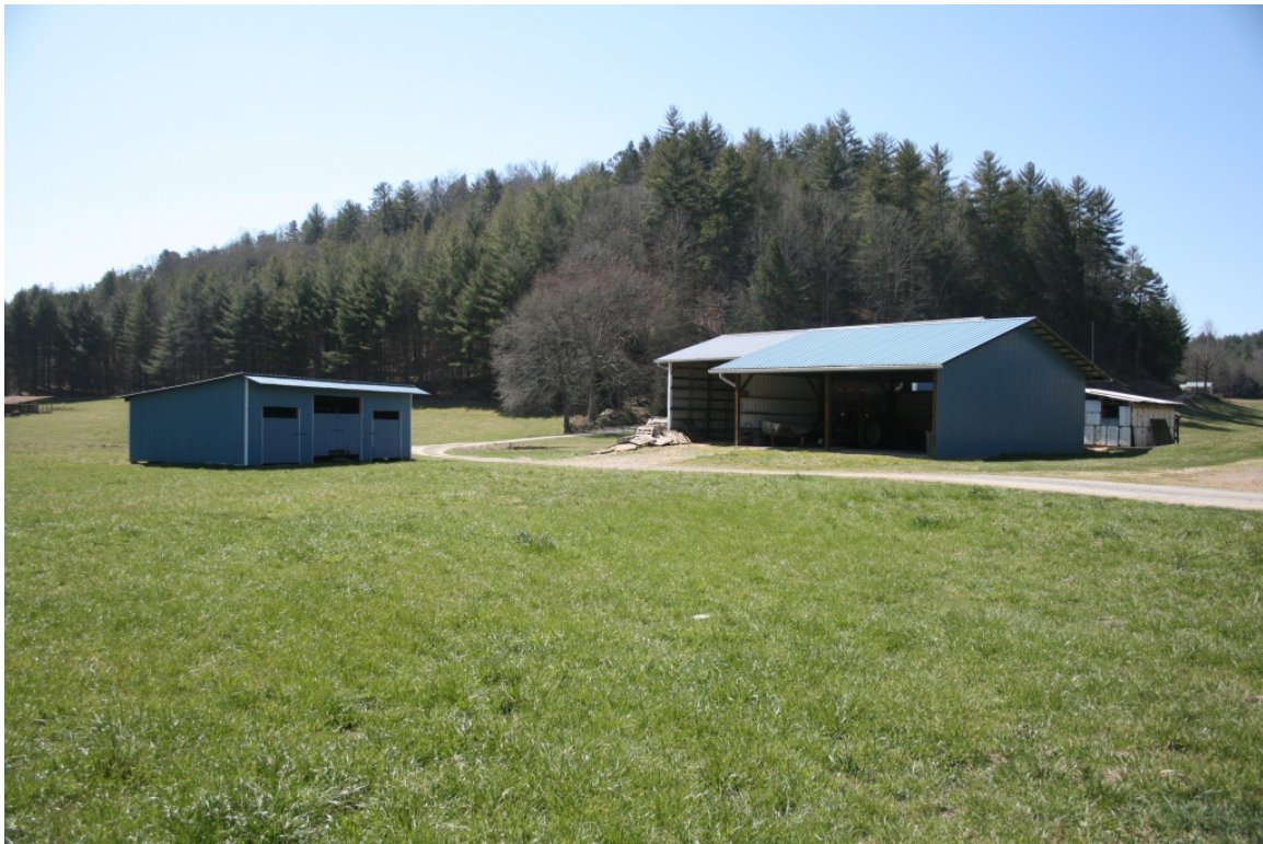
(L to R) Cow barn, hay barn, tractor shed, and brood house, view to southwest
