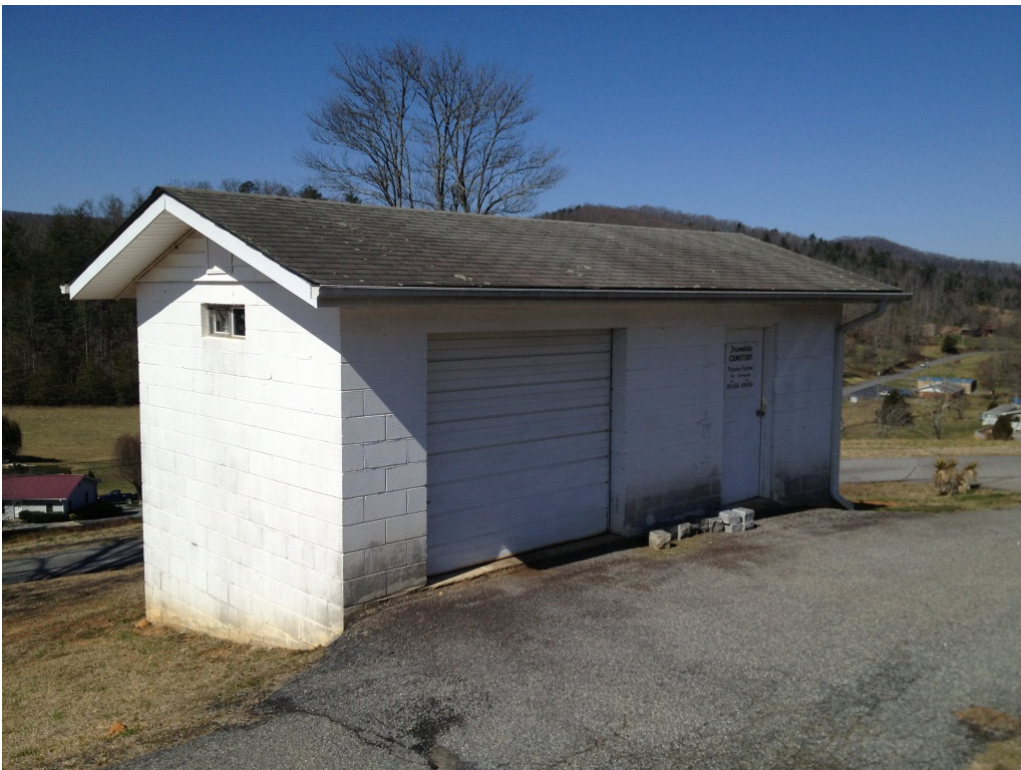
Maintenance building, oblique view to northwest
