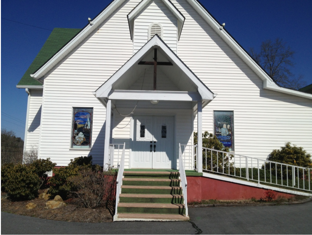
Friendship Baptist Church, façade, view to northwest
