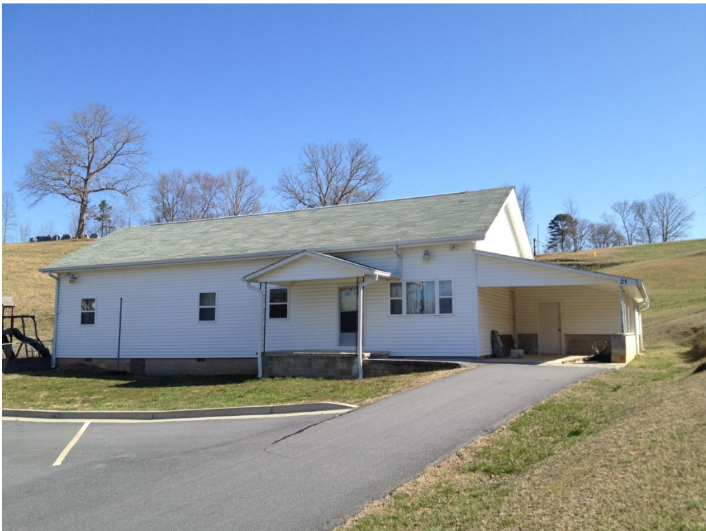
Friendship School (present-day Friendship Baptist Church Youth House), oblique front view to northeast
