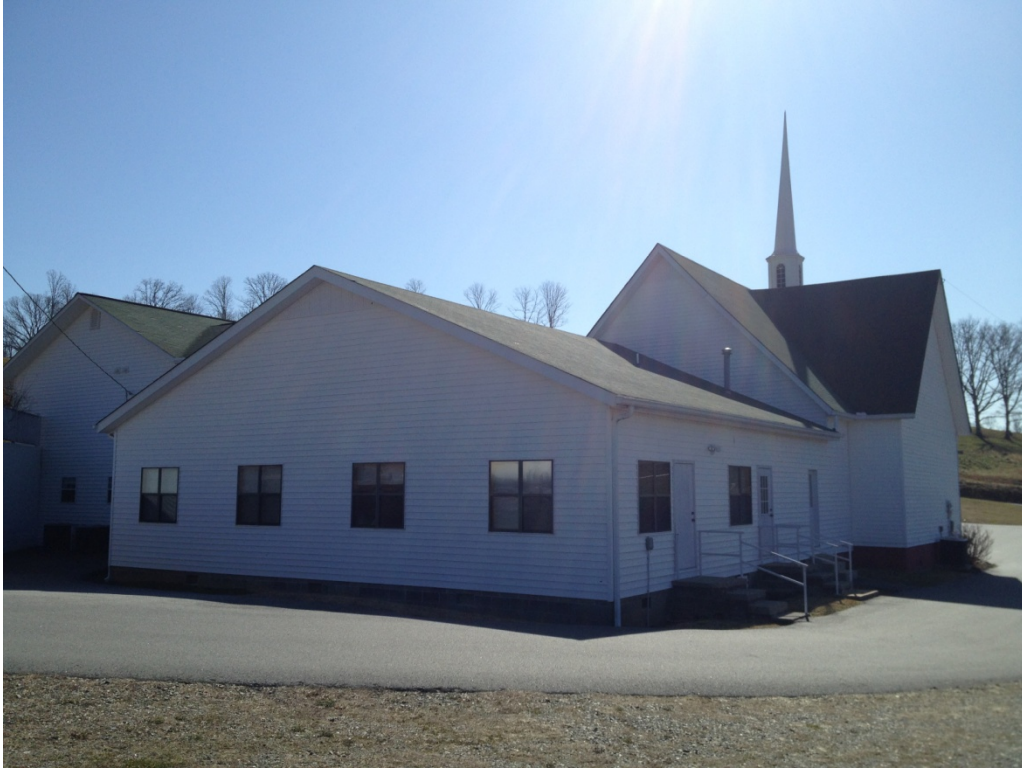
Friendship Baptist Church, oblique rear view to southeast
