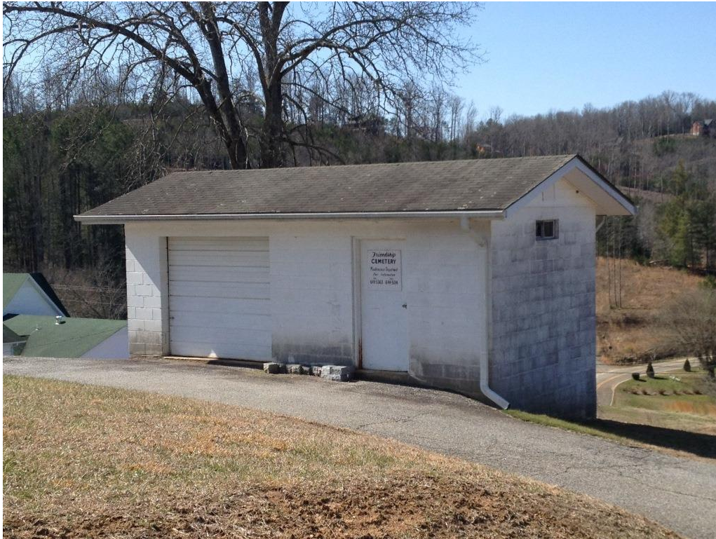
Maintenance building, oblique front view to south
